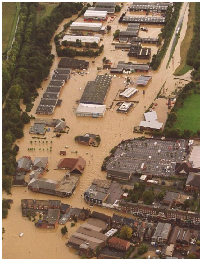
Flooding of the Uckfield Industrial Estate on 12 th October 2000. Courtesy of D. Charity, Solent News
